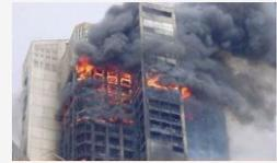
resistance, however, concrete structures must still be designed for fire effects and the behaviour of concrete structures in fire can be complex. Temperature rise causes a decrease in the strength and modulus of elasticity for both concrete and its steel reinforcement as well as the expansion of structural components and loss of structural integrity through cracking and spalling of concrete material.
